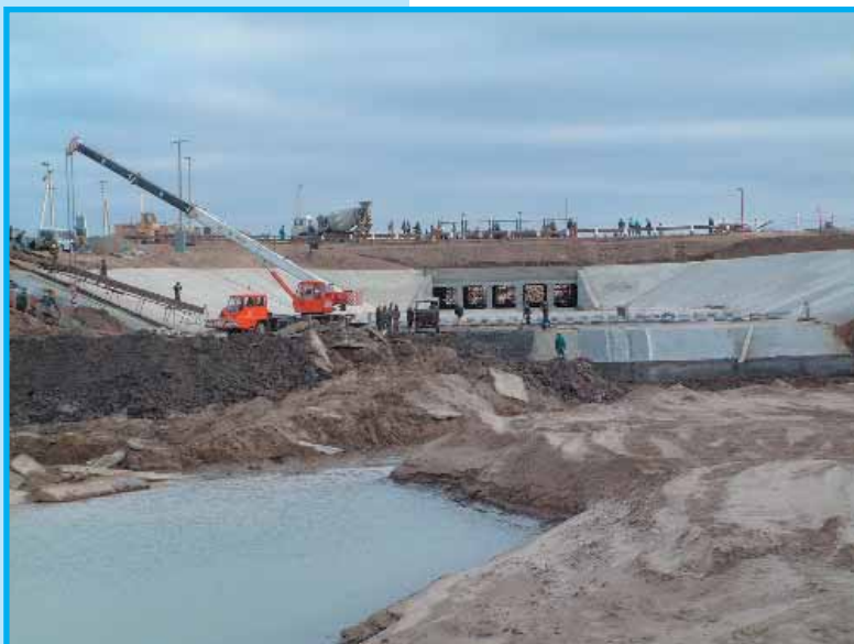
Last works on Aitek dam reconstruction, in the Karaozek area, operated by the Chinese Geo-engineering Corporation. The maximal flow in the Syrdarya will be raised from 300 m 3 /s to 700 m 3 /s.
